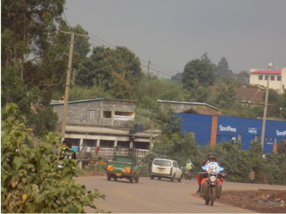
Figure 3: Some of the buildings alleged to be built over the former wetland outlet.
